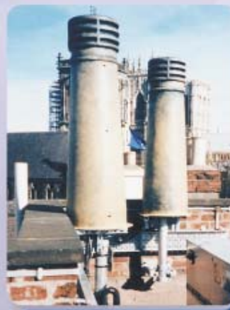
Antenna concealed in GRP chimney pots close to York Minister
